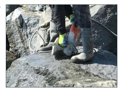
2. Circular saw used to make a second series of cuts perpendicular to first cuts (typically at 50mm centres).
