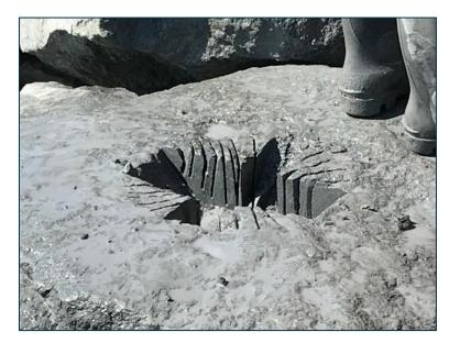
5. Breaker used to break out loose rock fragments and form dish/bowl shape approximately 300mm diameter with depth of approximately 150mm in centre.
